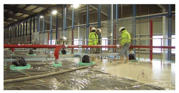
Highflow<sup>™</sup> S provides you with a high performance fast track solution to the construction of screeded floors.
