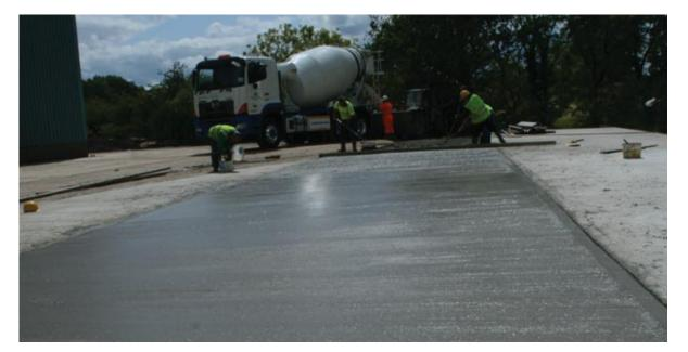
Highpave<sup>™</sup> is a range of fibre reinforced pavement grade ready-mixed concrete that reduce the errors associated with the use of conventional reinforcing methods.
