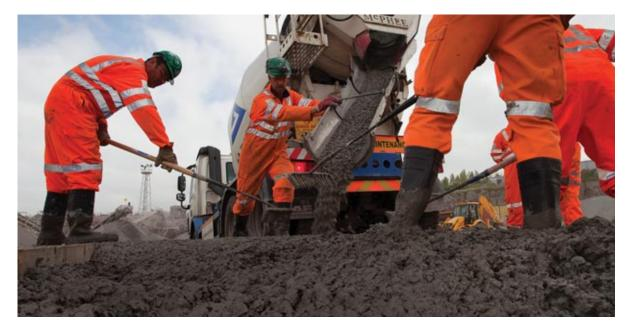
Emerald<sup>®</sup> is a range of concrete mixes that incorporate materials that are locally sourced where possible including secondary, recycled and reprocessed aggregates in addition to Portland Cement substitutes. Emerald<sup>®</sup> provides specifiers and contractors a fit-for-purpose concrete solution that has a reduced impact on the environment.
