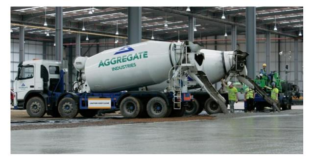
Extend<sup>™</sup> is a range of low shrinkage concrete designed to reduce joint frequency for both flatwork and structural applications thus offering improved in-service performance and reduced construction costs.
