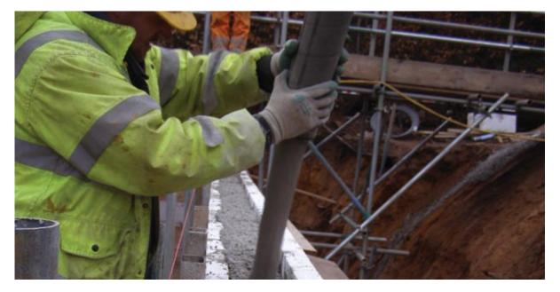
Widely used in the USA, Canada and Continental Europe, ICF (Insulating Concrete Formwork) is a relatively new UK building technique which involves a series of hollow expanded polystyrene blocks into which ICF-Crete<sup>®</sup> is poured. The system combines the inherent strength of concrete with the excellent thermal insulation properties of polystyrene to produce cost effective and durable structures.
