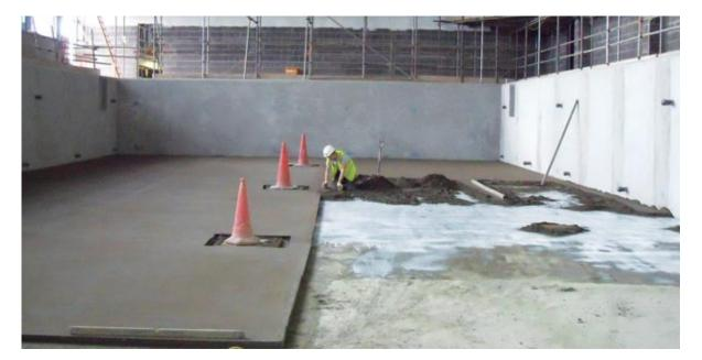
A range of cement bound products produced under factory conditions and available in a range of grades from C5 to C30.
