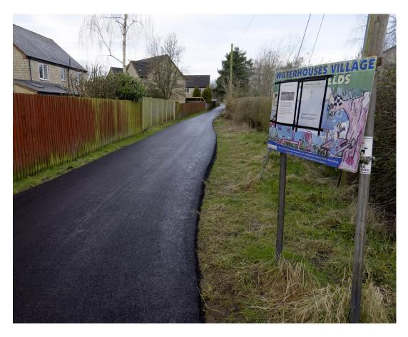
Additionally, 40 tonnes of AC10 close graded surface course material was laid.
