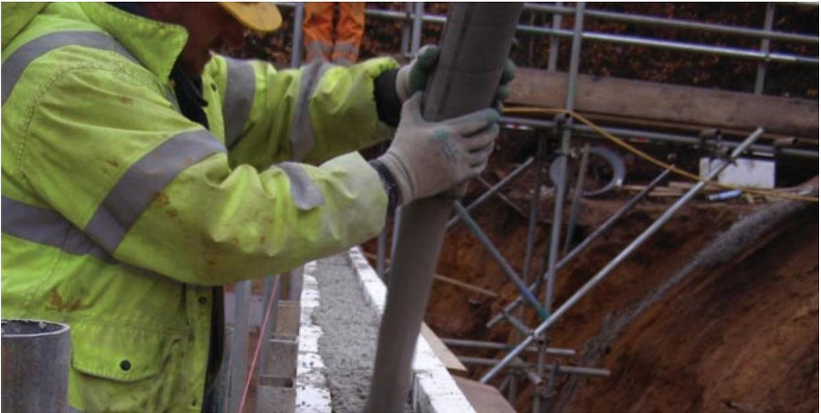
Widely used in the USA, Canada and Continental Europe, ICF (Insulating Concrete Formwork) is a relatively new UK building technique which involves a series of hollow expanded polystyrene blocks into which ICF-Crete® is poured. The system combines the inherent strength of concrete with the excellent thermal insulation properties of polystyrene to produce cost effective and durable structures.
