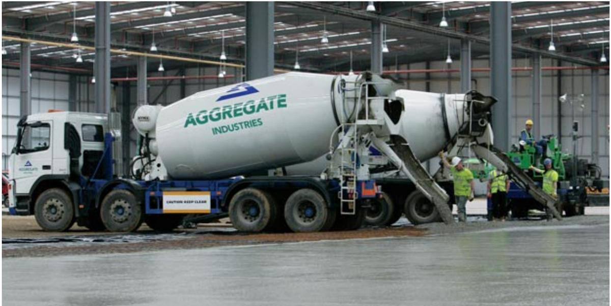
Extend™ is a range of low shrinkage concrete designed to reduce joint frequency for both flatwork and structural applications thus offering improved in-service performance and reduced construction costs.
