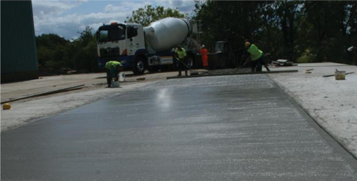
Highpave™ is a range of fibre reinforced pavement grade ready-mixed concrete that reduce the errors associated with the use of conventional reinforcing methods.
